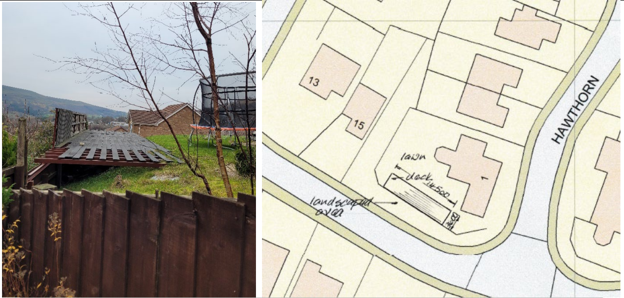
Fig 1.5 & 1.6 - Extent of decking to be retained, from within the garden and plan view.
