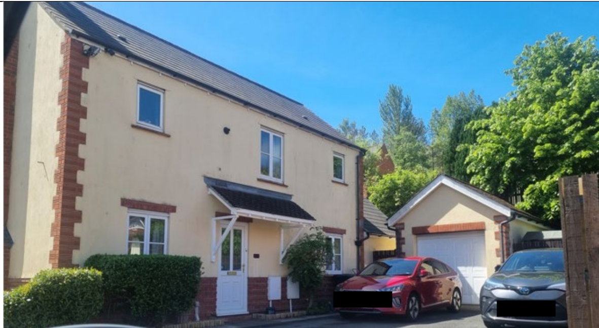
Fig 5. View of principal elevation, from the north
