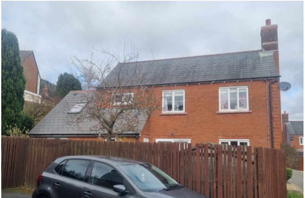
Fig 4. View from Village Lane, approaching from the South
